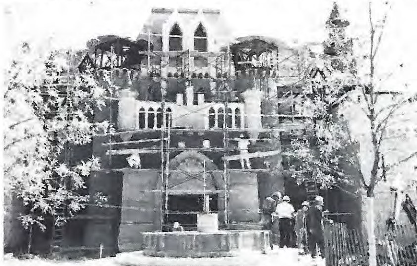
The medieval castle with stonemasons working on the facing.
