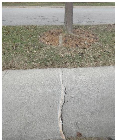
**Figure 2** Example of a tree root lifting and cracking a sidewalk.
