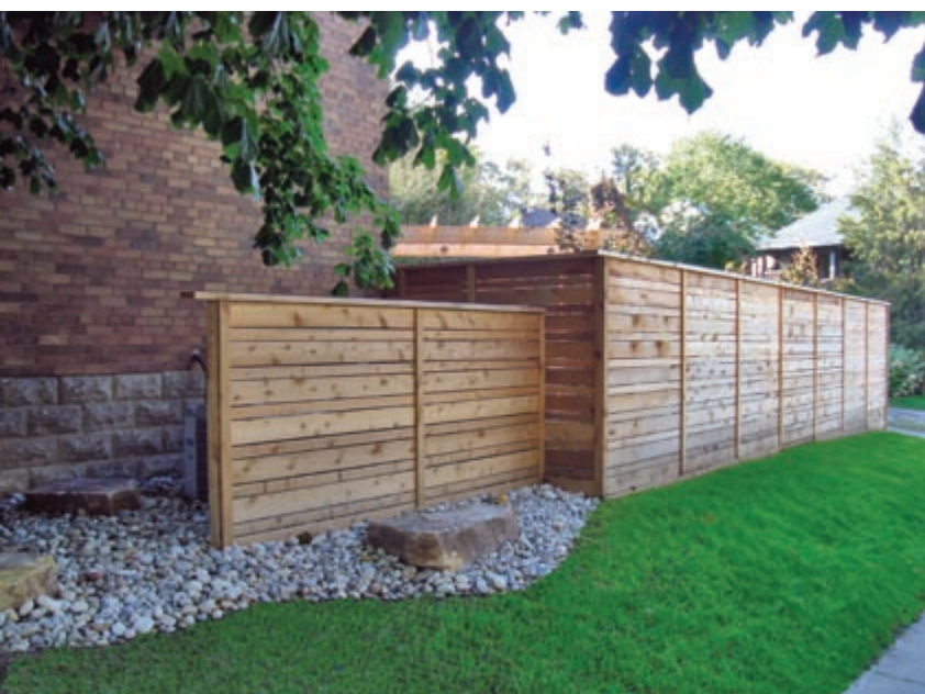
By extending and modifying the fence on this corner lot, the designer hid an unsightly air conditioning unit, yet kept it easily accessible for servicing. Larger stones situated in the bed of river pebble create the illusion of a dry stream. The alternate wide and narrow horizontal boards of the fence ensure both privacy, yet allow some light to pass through into the concealed patio. Sacred Space Landscape & Design
